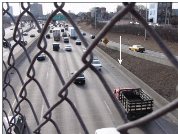
Figure 7: Southward view from oblique overpass showing approximate area of impacts and final rest for both vehicles; Note: arrow indicates suspected impact location between one of the vehicles and longitudinal barrier (case photo #11a)
