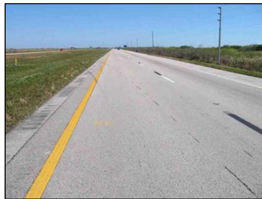
Figure 3 - CCW tire marks leading to road departure.
