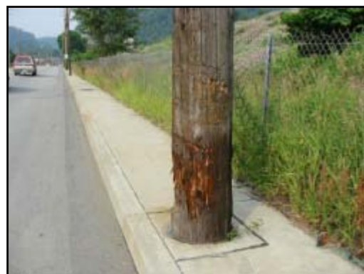
Figure 3. GMC's impact with utility pole.
