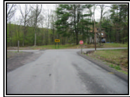
Figure 2. View of T-intersection looking south
