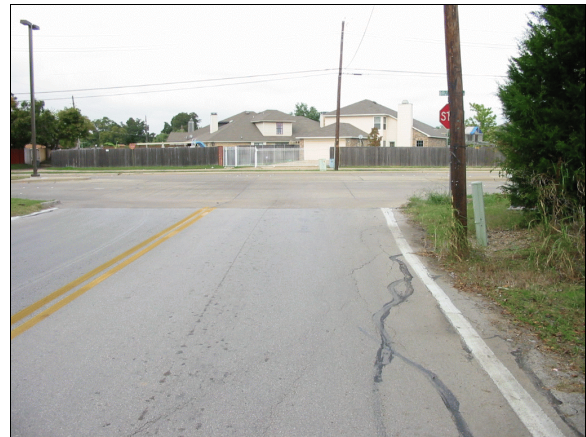
Figure 1: Case vehicle's northward travel path approaching Tee intersection (case photo #01)
