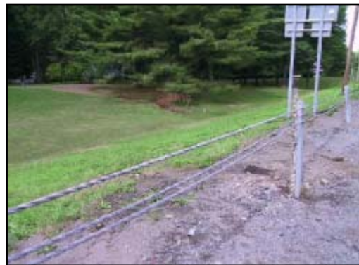
Figure 5. Volvo guardrail rail impact.
