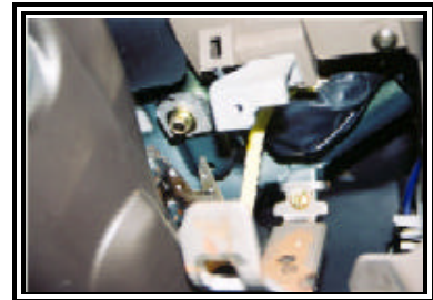
Figure 8. Right shear bracket separation.
