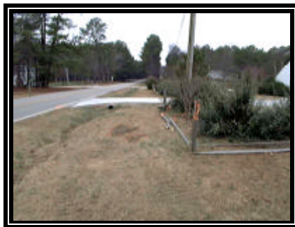
Figure 6. Wood fence impact and utility pole (replaced)
