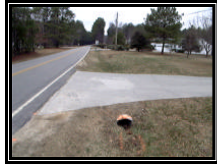
Figure 4. Point of impact with the culvert
