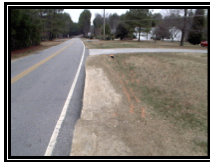
Figure 3. Point of roadway departure
