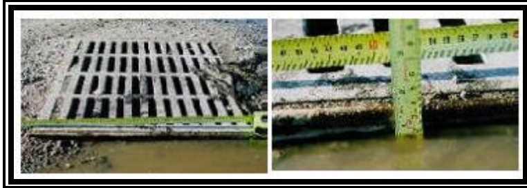
Figure 2. North view of struck sewer grate and associated height measurement.
