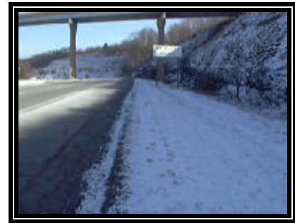
Figure 2. Approach view showing the point of roadway departure
