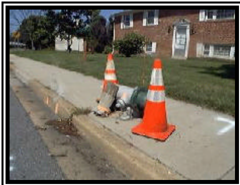
Figure 2. Struck fire hydrant (foreground) and mailbox post (background).
