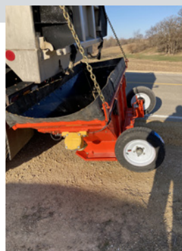
Jones County's hopper improved shoulder maintenance.
