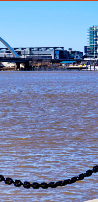
The new Frederick Douglass Memorial Bridge in Washington, DC, is the city's largest ever public works project.
