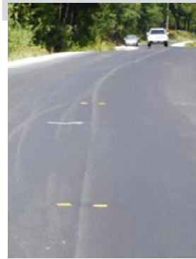
Thermoplastic centerline markings improve visibility and safety.
