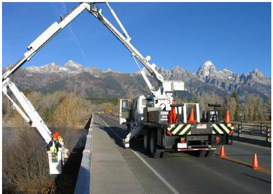
Inspectors use a bucket truck on the Snake River Bridge in Grand Teton National Park.
