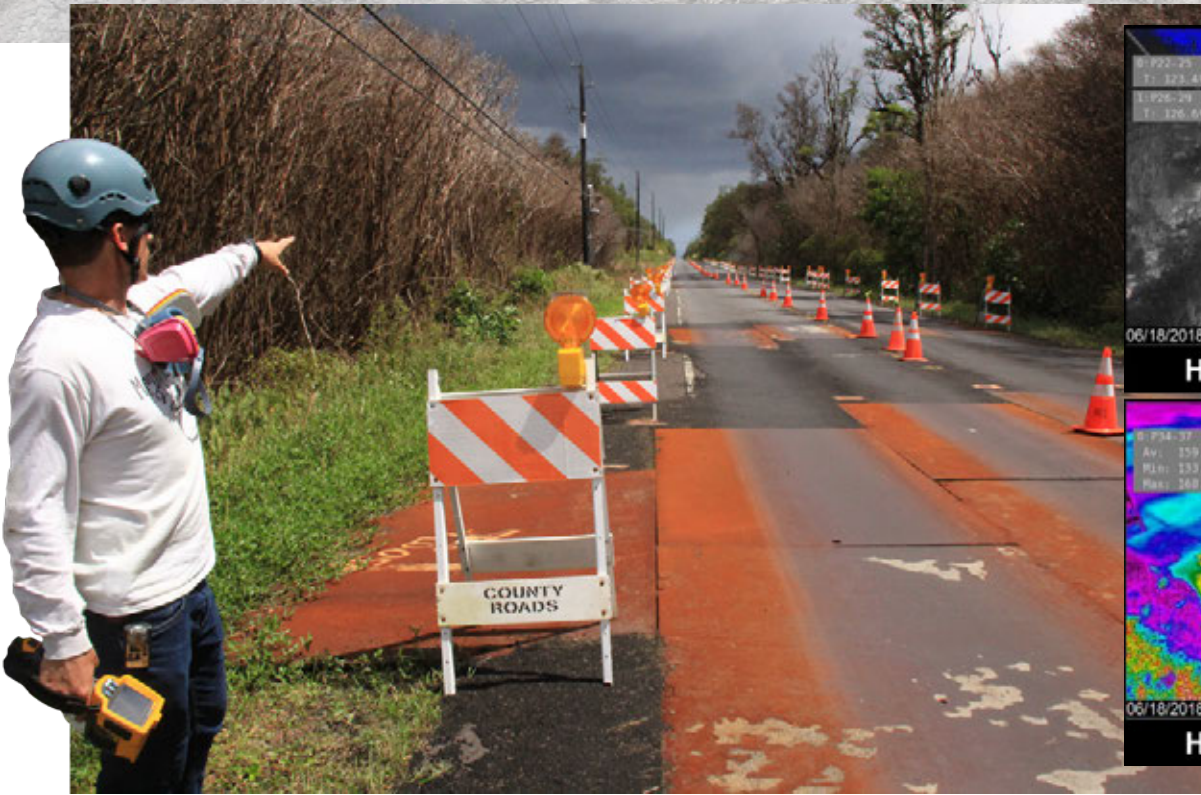
Field crews track activity in and around Leilani Estates in June 2018, including observations from cracks near Route 130, shown here with plates installed on the roadway.
