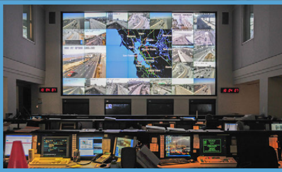
Traffic management centers like this one in California are the nerve centers of highway management.
