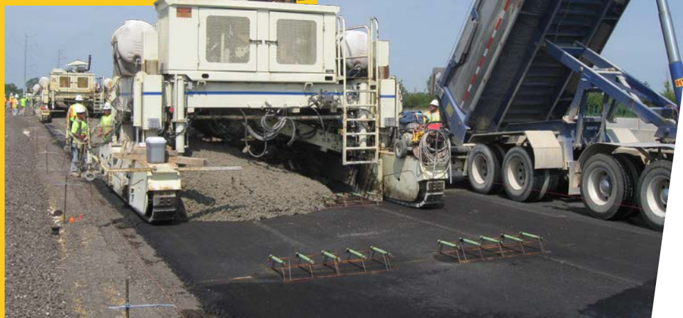
A construction crew pours fresh concrete on an asphalt base during construction of a jointed plain concrete slip-formed pavement.
