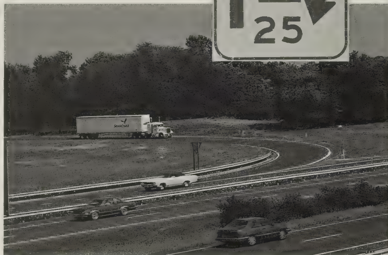
Despite the use of warning signs, truck rollover on curved exit ramps is still a significant problem.
