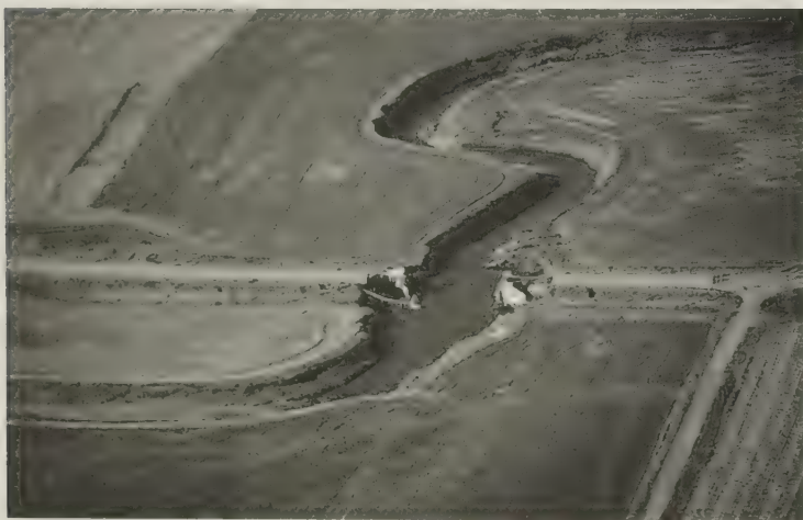
Although there were no major bridge failures along the Mississippi and Missouri Rivers during the great flood of 1993, long-term stream stability problems on tributaries caused damage to several bridges. At top, lateral migration of the Nemaha River channel in Nebraska resulted in the collapse of a bridge on state Route 8. At bottom, the bridge over Brushy Creek on Iowa state Route 71 is a classic example of failure caused by abutment scour.
