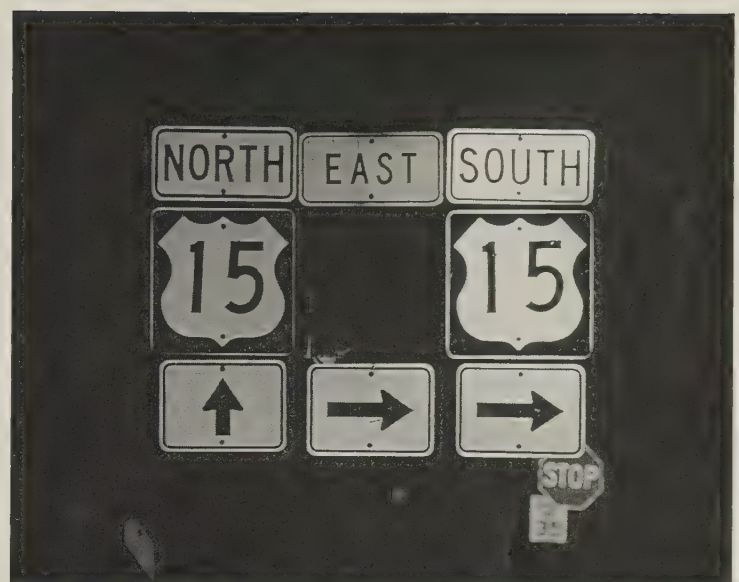
Signs with poor retroreflectivity cannot be easily seen at night and in adverse weather conditions.
