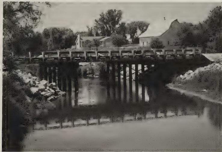
The Piney Creek Bridge is a stress-laminated timber bridge in Richland Center, Wisc.
