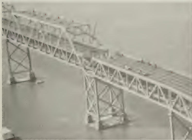
Figure 1.—Loma Prieta: vital transportation link closed.
