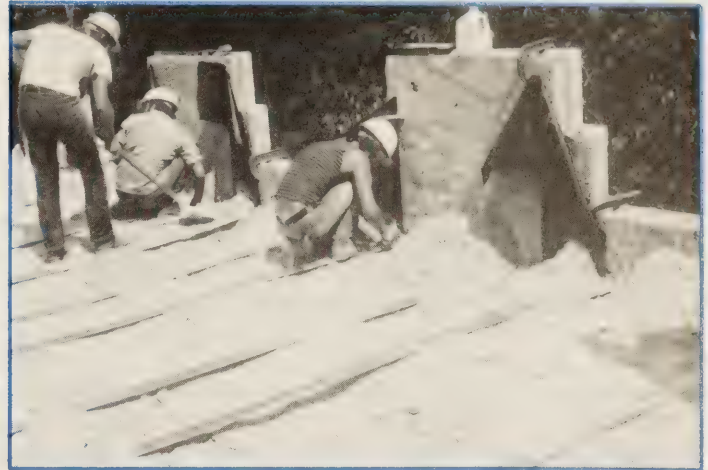
Figure 5.—Placing the major components of a reinforced soil structure.
