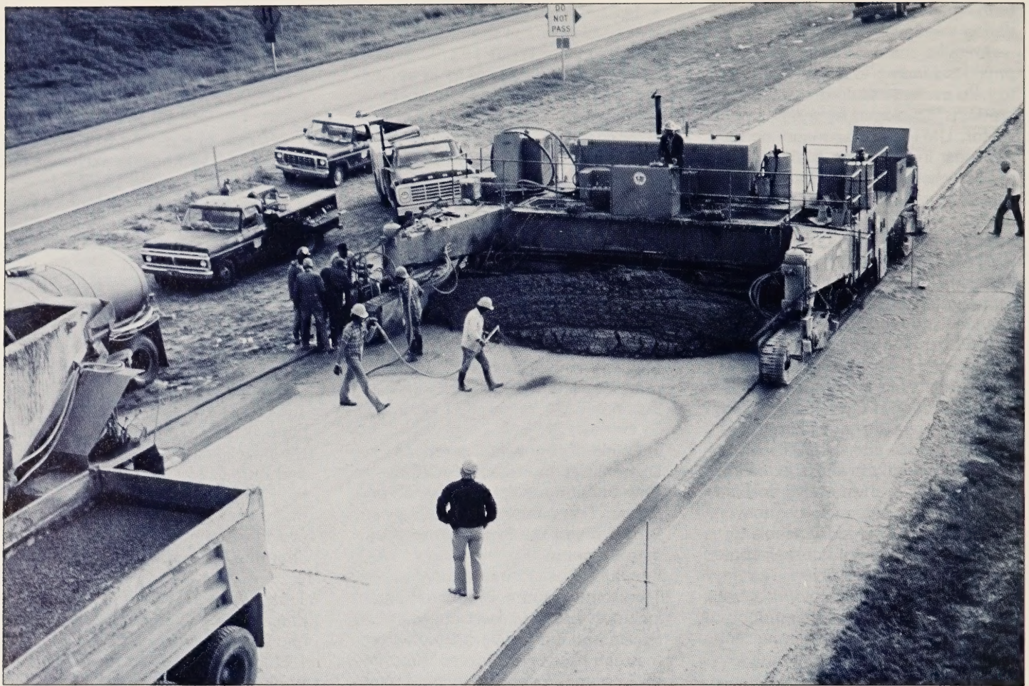
Figure 2.—A thin-bonded concrete overlay containing polypropylene fibers is one of the features being evaluated under the Experimental Projects Program.
