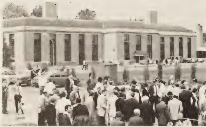
The Herbert S. Fairbank building is part of the Turner-Fairbank Highway Research Center in McLean, VA.
