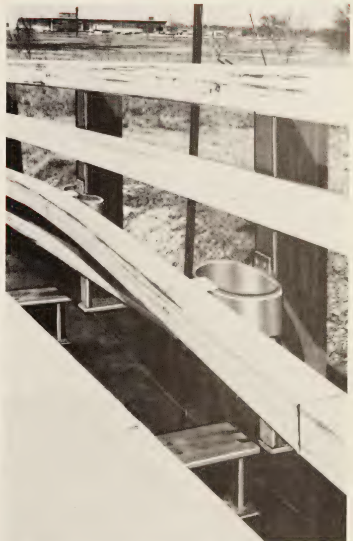
Collapsing ring, heavy bridge rail design. (3)
