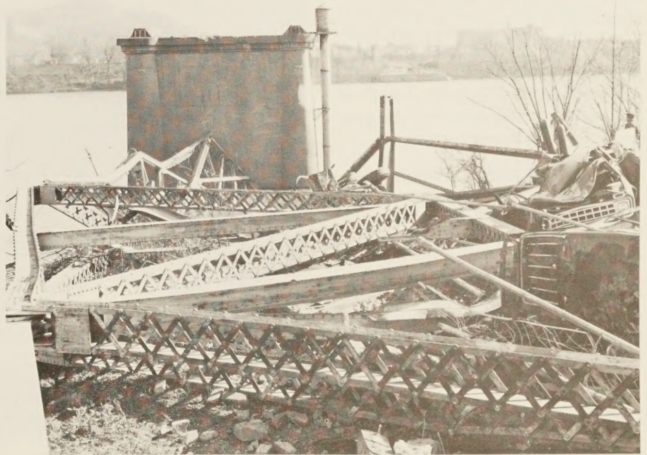
Figure 3. — Silver Bridge after collapse.
