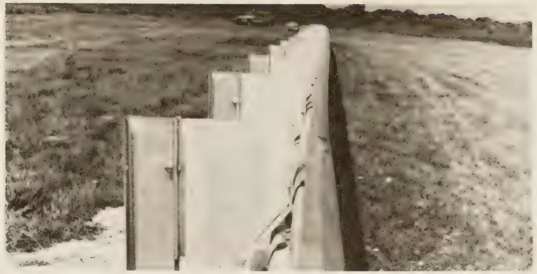
Figure 14. —Modified three beam guardrail after test with Honda Civic.
