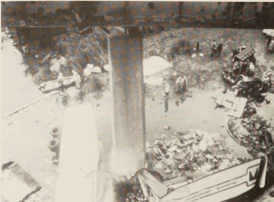
Figure 6. —Mianus River Bridge after collapse.
