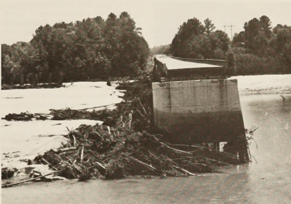
Figure 7. — Typical bridge damage from flooding.
