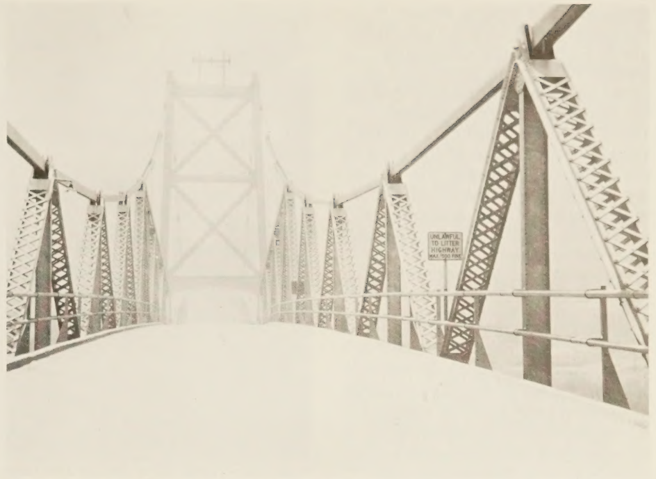
Figure 2. — Silver Bridge, Point Pleasant, West Virginia.
