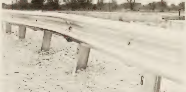
Figure 15. —Strong post "W" beam guardrail after test with Honda Civic.
