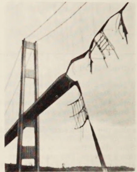
Figure 1.—Tacoma Narrows Bridge collapse.
