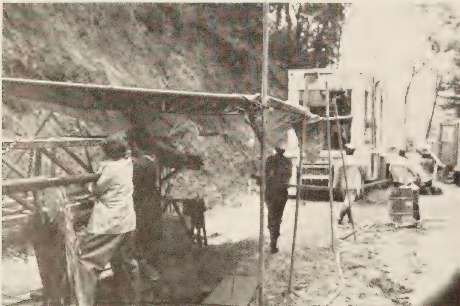
Figure 11. —Probe withdrawal from water-filled borehole at the Cumberland Gap Tunnel site.
