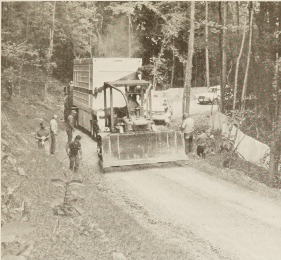
Figure 5.—The MUSE is manipulated into position for logging an experimental borehole at the Cumberland Gap Tunnel site.
