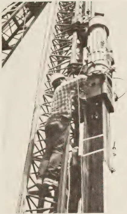
Figure 2. —Pile analyzer equipment used to monitor pile installation.
