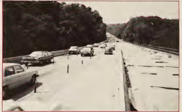
Figure 2. — Examples of vertical tubes used on the George Washington Memorial Parkway.
