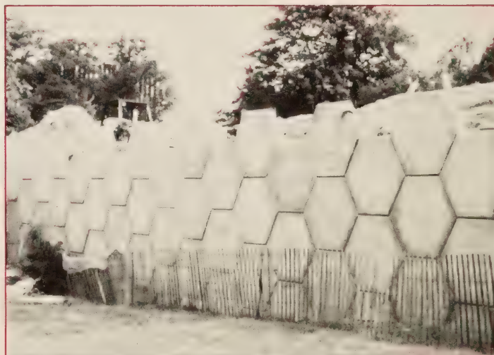
(b) Nearly completed front facing of Reinforced Earth wall.
