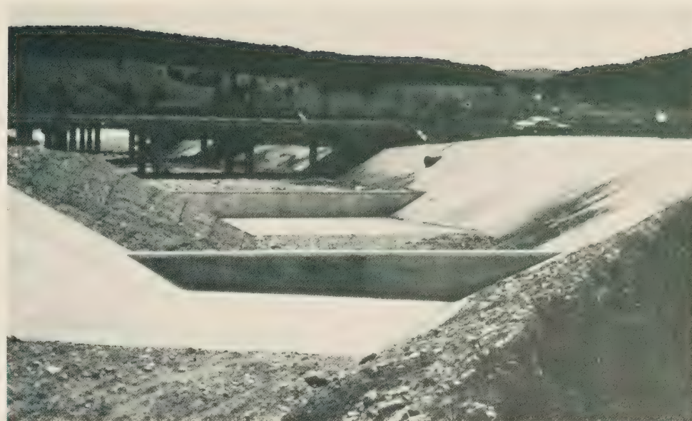
Figure 7.—Series of check dams to mitigate a serious degradation problem.
