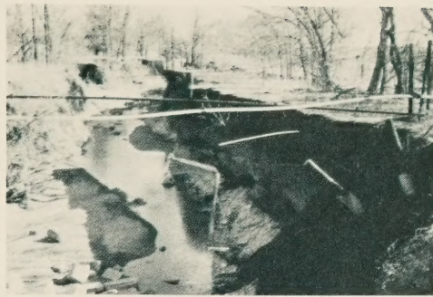
Figure 4.—Extreme case of degradation resulting in bank erosion (both banks), slumping, and debris problems.
