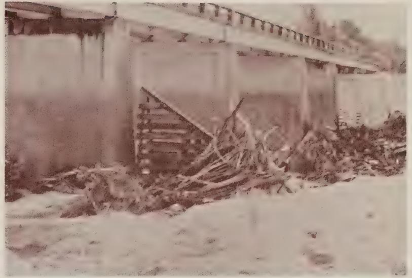
Figure 7.—A debris fin (foreground) and a debris crib (last pier).
