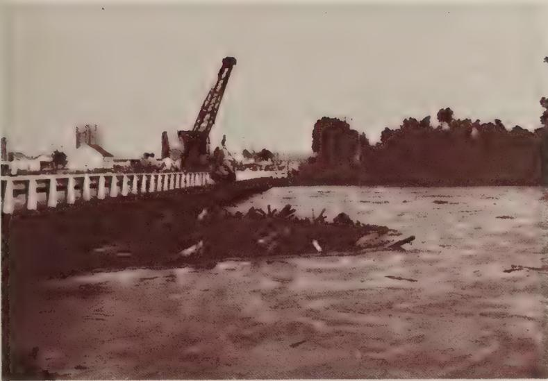
Figure 6.—Crane being used to remove hazardous debris.
