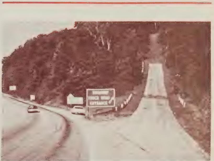
Figure 3.—Combination arrester bed and gravity ramp.
