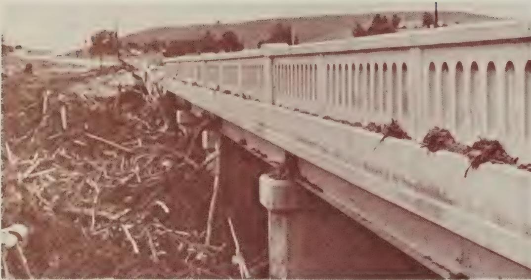
Figure 4.—Massive debris pile-ups may constrict flood flow and result in scour at the bridge pier. Note damaged deck at the far end of the bridge.
