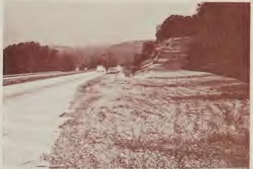
Figure 2.—Arrester bed ramp being constructed.
