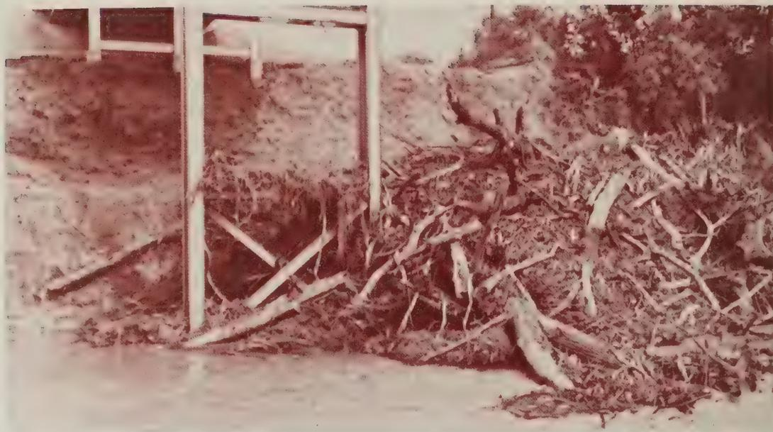
Figure 2.—Massive vegetation debris accumulation on a bridge pier.
