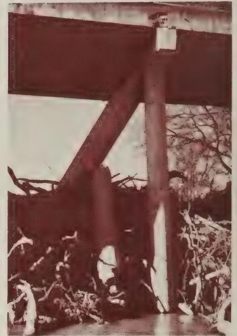
Figure 5.—The lateral forces of water against a large debris accumulation caused the destruction of this bridge pier.
