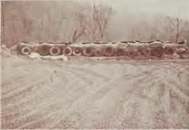
Figure 4.—Arrester bed ramp with attenuator.
