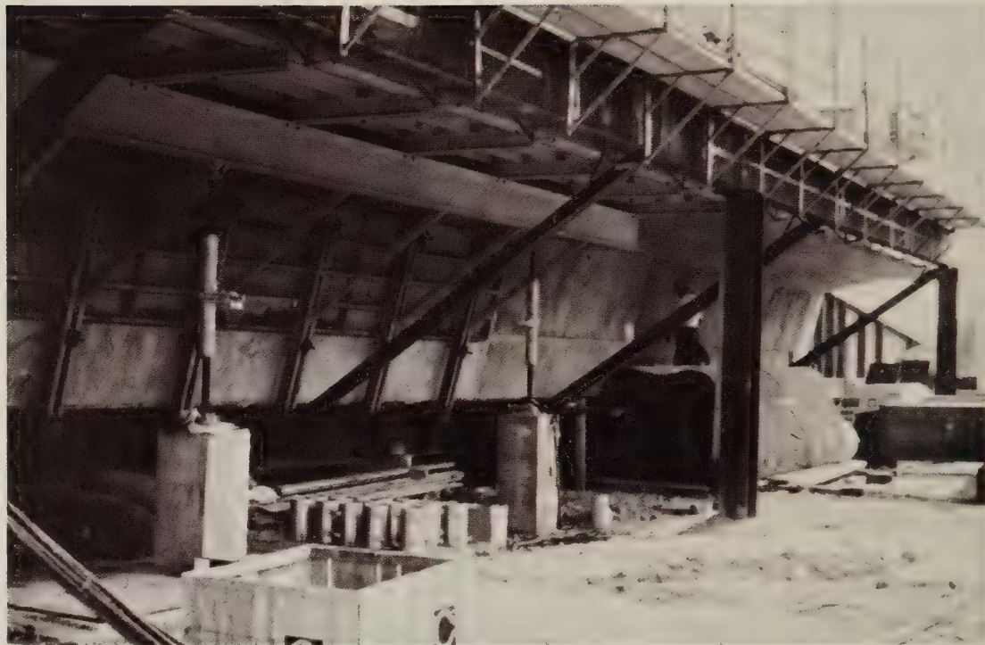
Figure 3.—Wabash River bridge under construction.
