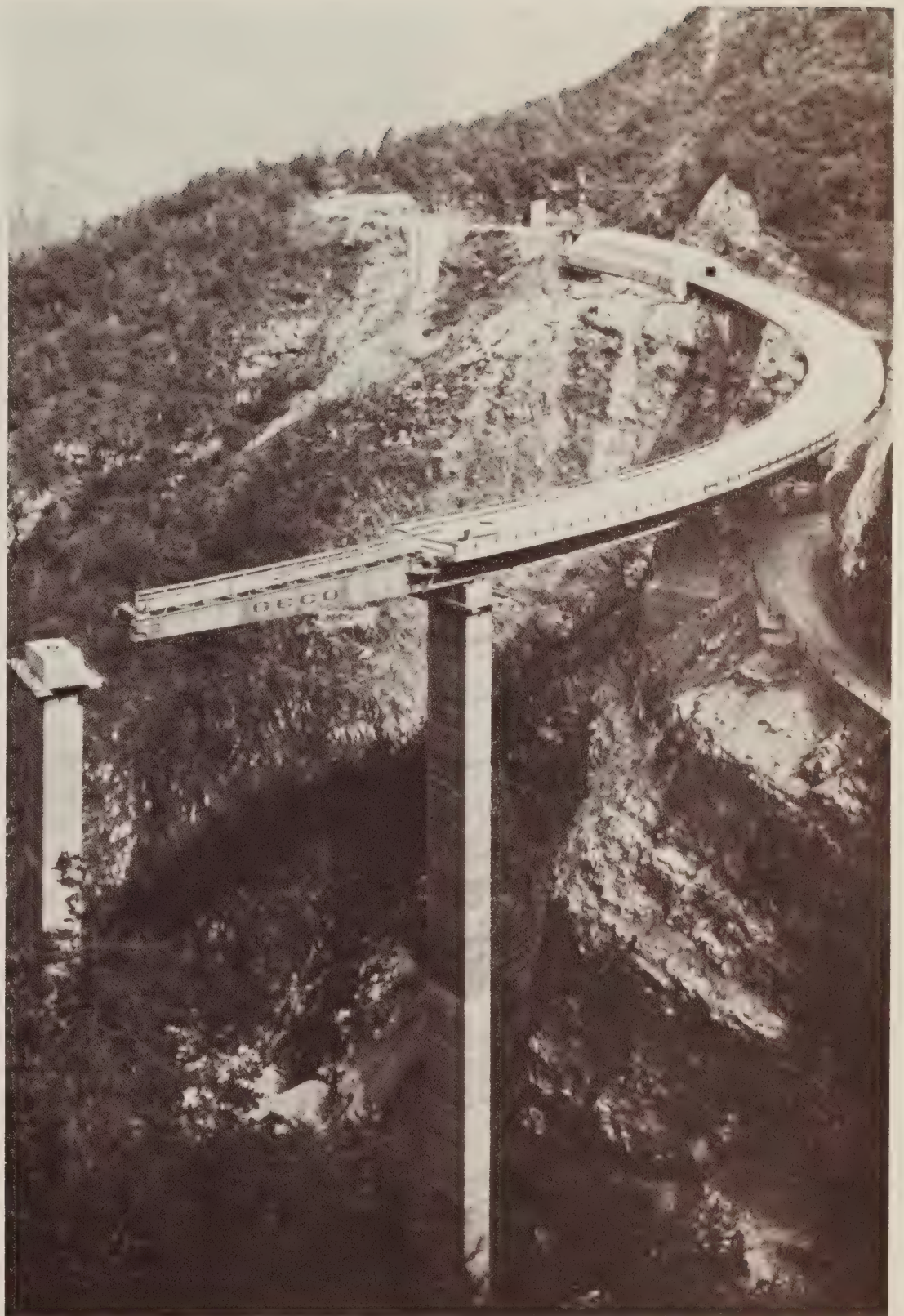
Figure 2.—Incremental launching of bridge superstructure.
