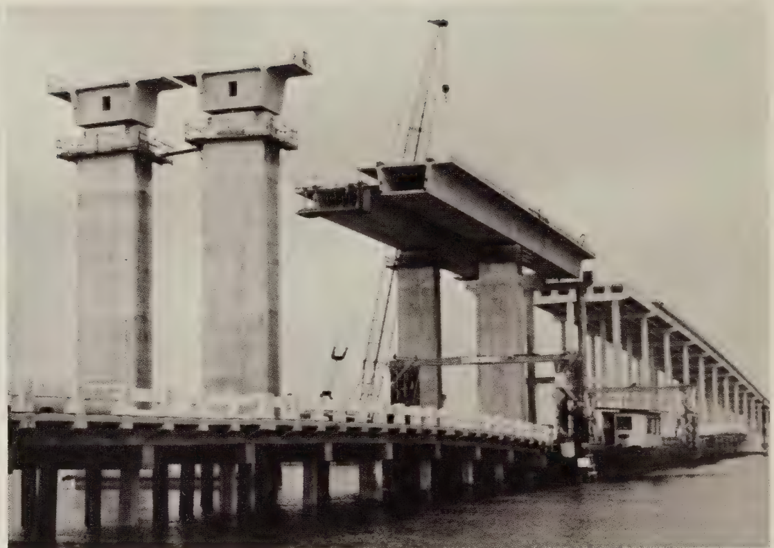
Corpus Christi Bridge under construction.
