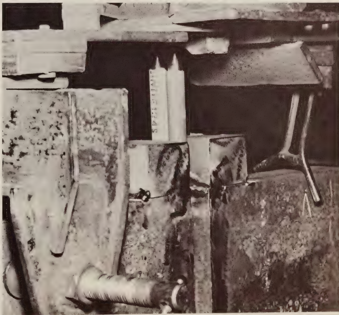
Figure 2b.—Double guide tube used in 3-in (76 mm) thick joint (note flux coating on guide tubes).
