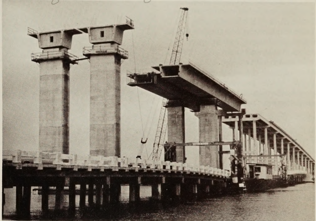
Corpus Christi Bridge under construction.
