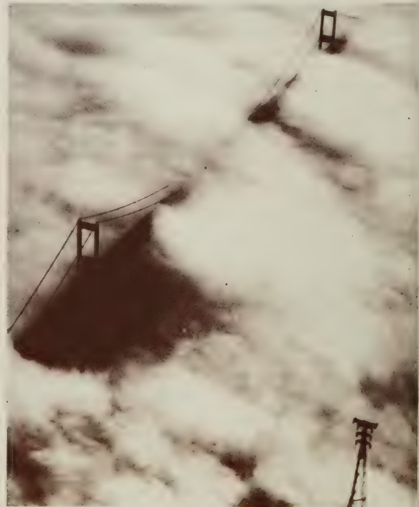
Figure 2.—The Severn Bridge in Great Britain under patchy fog conditions.
