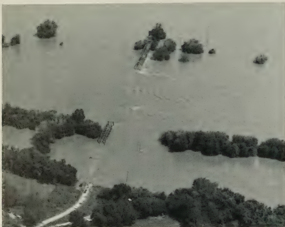
Flood damage caused by Hurricane Agnes in June 1972 at Cartersville, Va. Note the pins remaining in place while the superstructure and roadway surface in the middle channel are lost.
