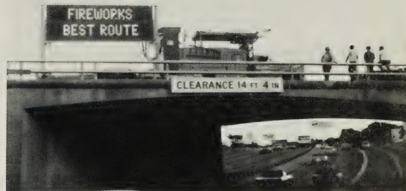
Figure 4.—Experimental trailer mounted motorist information sign used in a Texas research study.
