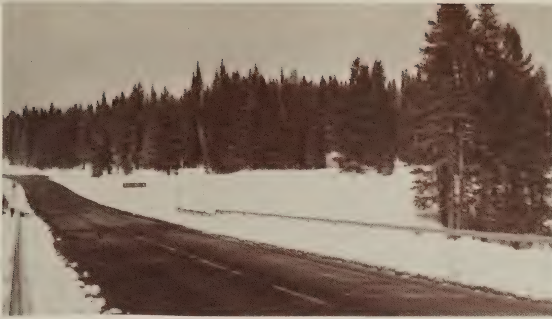
Figure 8.—Test site—California State Route 89, 5 miles north of Truckee, Calif.
