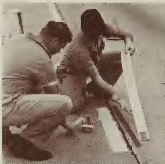
Figure 4.—Taped stripe prior to installation.
