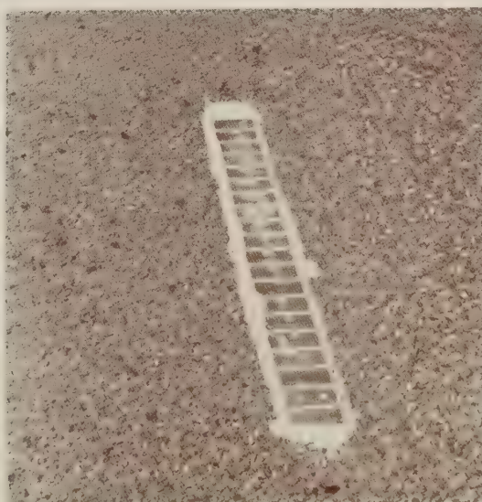
Figure 3.—Complete stripe installed on the road surface.
