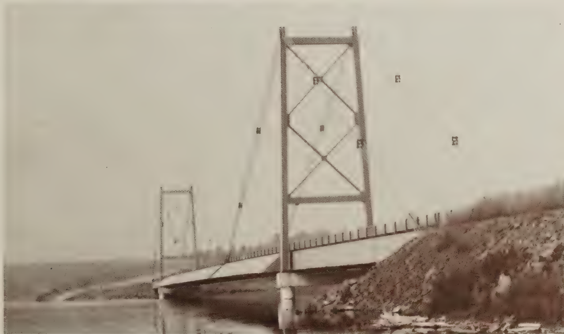
Figure 6.—Modified Long's Creek Bridge.
