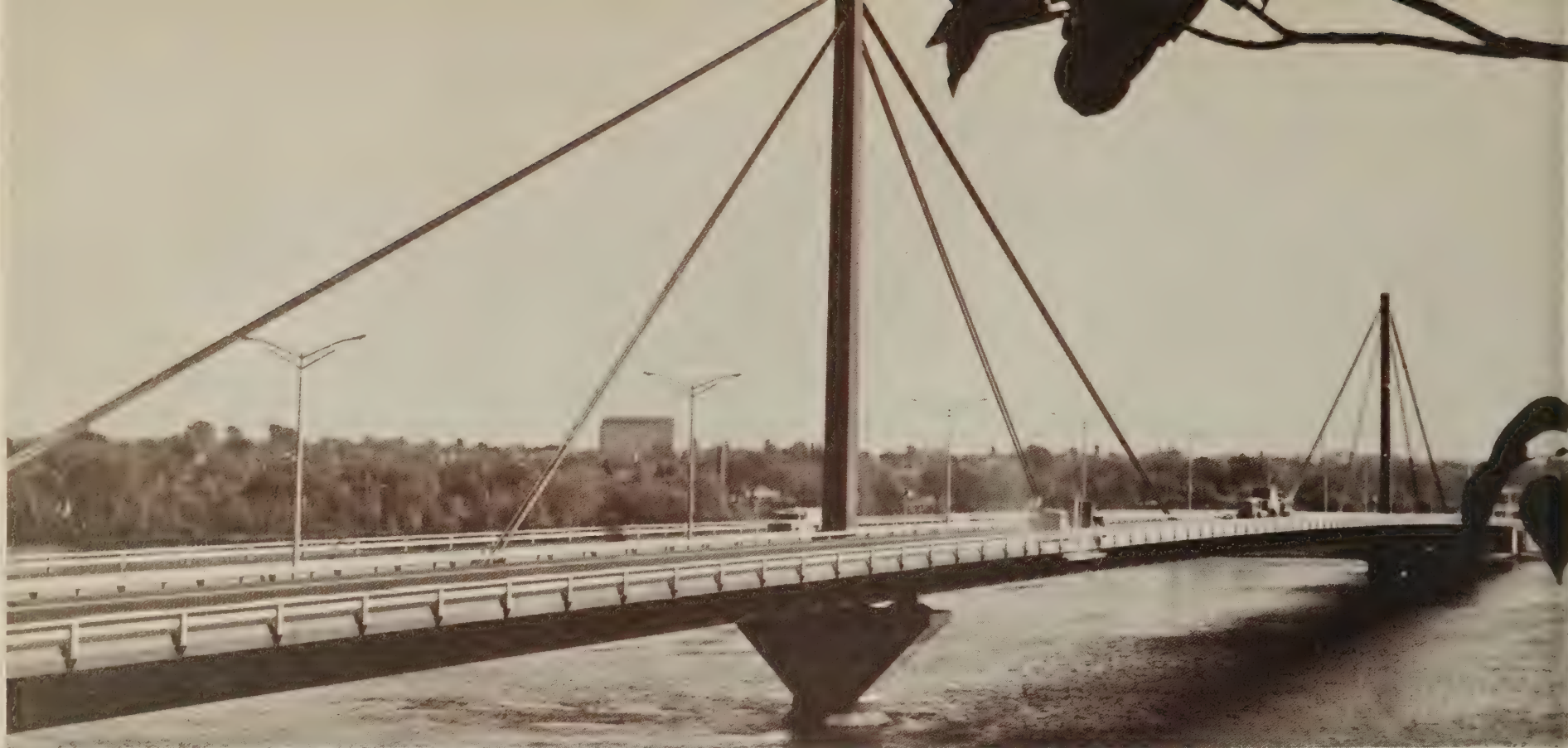
Papineau Bridge, Montreal, Canada.
