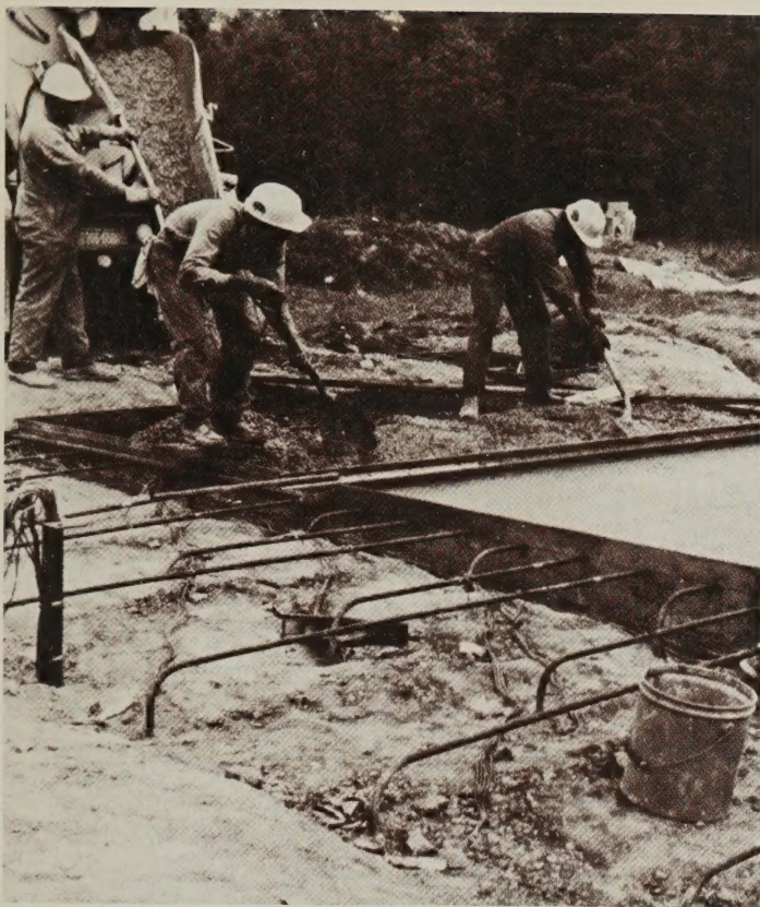
Figure 3.—Pouring earth heat pipe slab.
