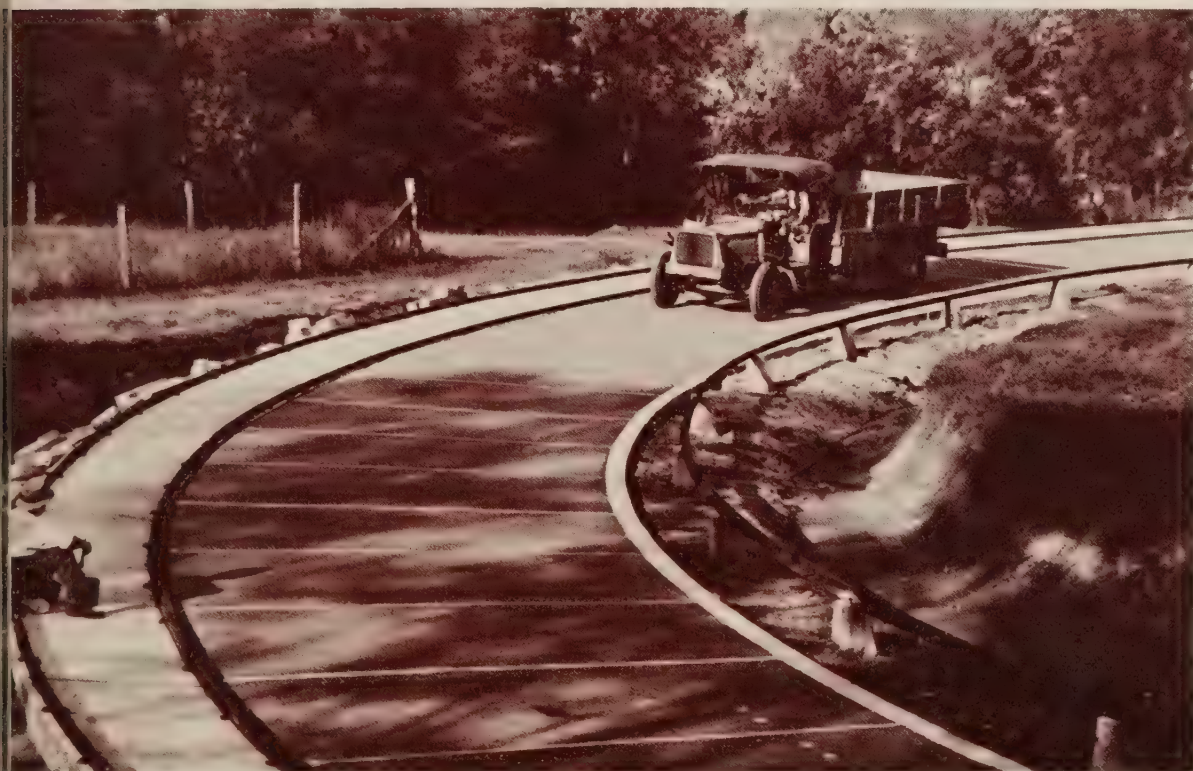
Figure 5.—View of the circular track at Division of Tests site in Arlington, Va., in early 1920's. This track was used to establish a number of the principles of pavement and base course design and was probably the first accelerated testing system used in the United States. "Traffic" was provided by the truck driven continually in circles for 8 hours each day. Note the solid tires on the truck.
