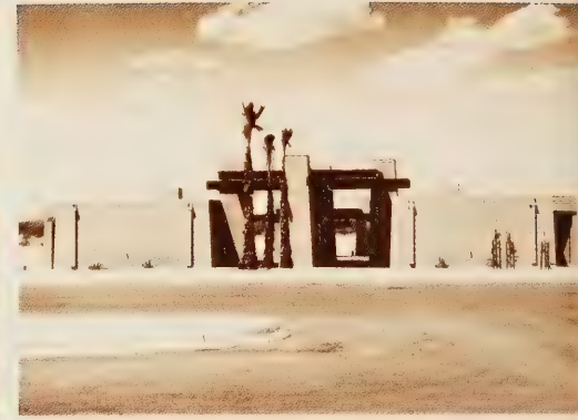
Figure 3. — Building with historical architectural treatment.
