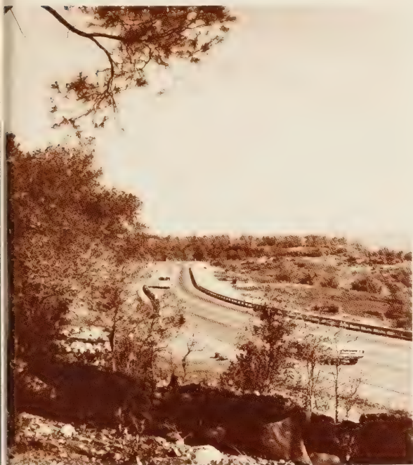
Figure 3.—Natural vegetation provides beauty, reduces maintenance costs, and eliminates driver monotony.
