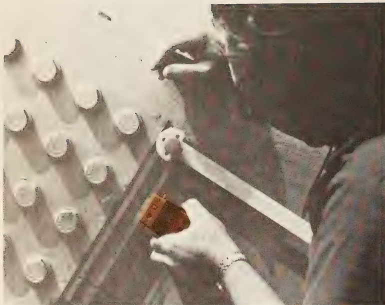
Figure 8.—Typical inspection using ACD for detecting cracks between bolt holes under cover plate.
