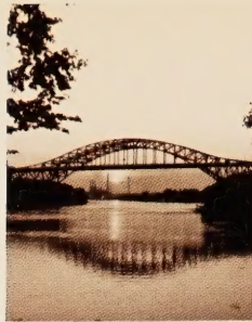
Piscataqua River Bridge on I-95 between Kittery, Maine, and Portsmouth, N.H. (Photo courtesy of the Maine Department of Transportation and the New Hampshire Department of Public Works and Highways.)
