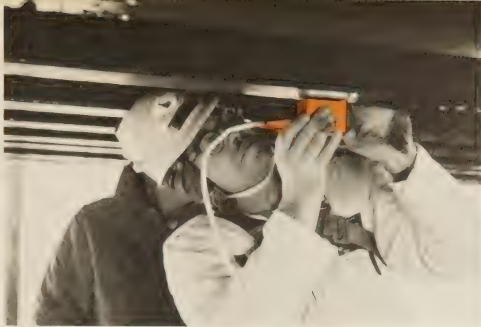
Figure 10.—Selected views of Idaho State Highway Department personnel inspecting I-beams of American Falls Dam Bridge in February 1973 (temperature 14°-30°F).
