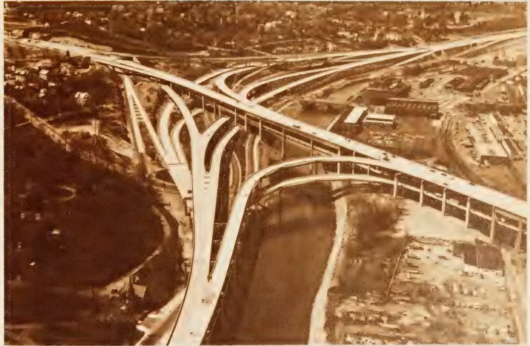
Figure 1.—Highspeed urban expressway.
