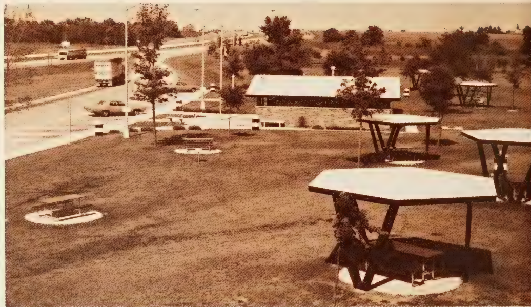
Figure 4. — Rest area with picnic tables, shelters, and cooking grills.
