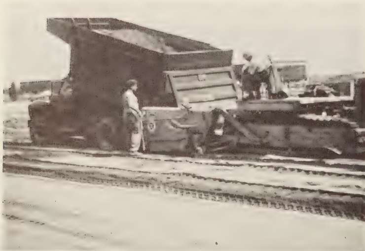
Figure 12.—Stabilized sulfate waste being placed by a material spreader.
