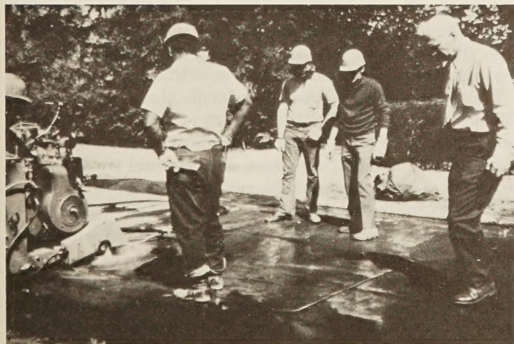
Figure 6.—Self-propelled saw cutting loop slot.
