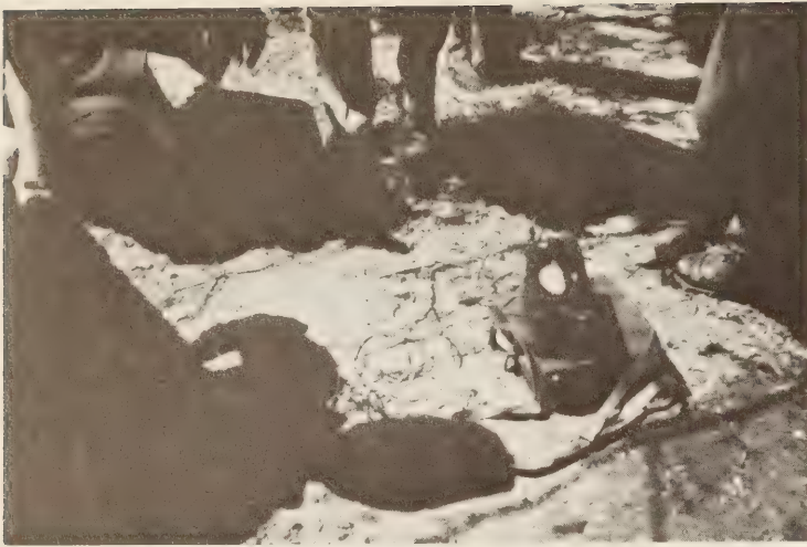
Figure 12.—Use of Megger meter.
