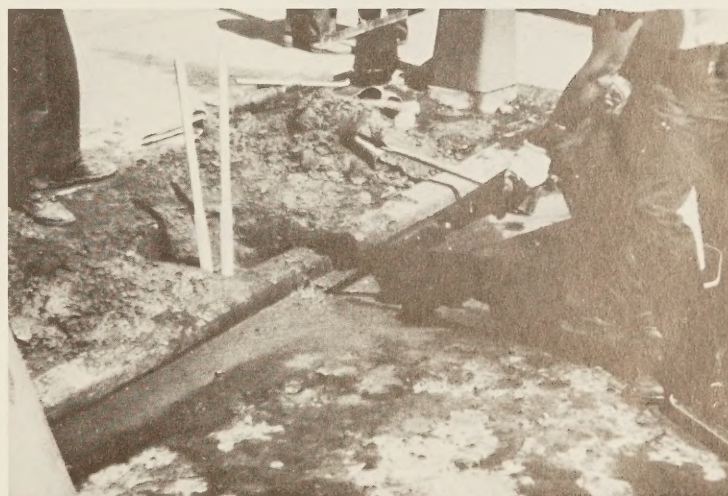
Figure 8.—Drill for boring hole through curb.
