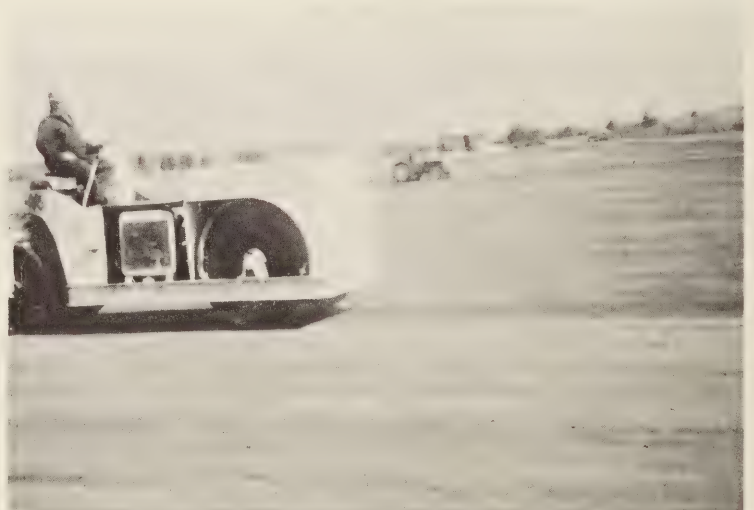
Figure 13.—Compacting stabilized waste parking area, Dulles International Airport.
