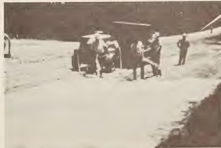
Figure 9.—Regraded section being covered with Fiberglas roving.
