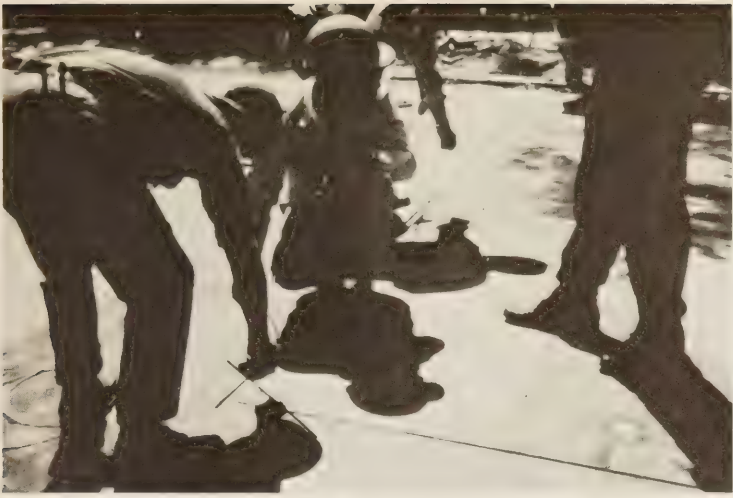
Figure 17.—Protective plates over sawed slots.
