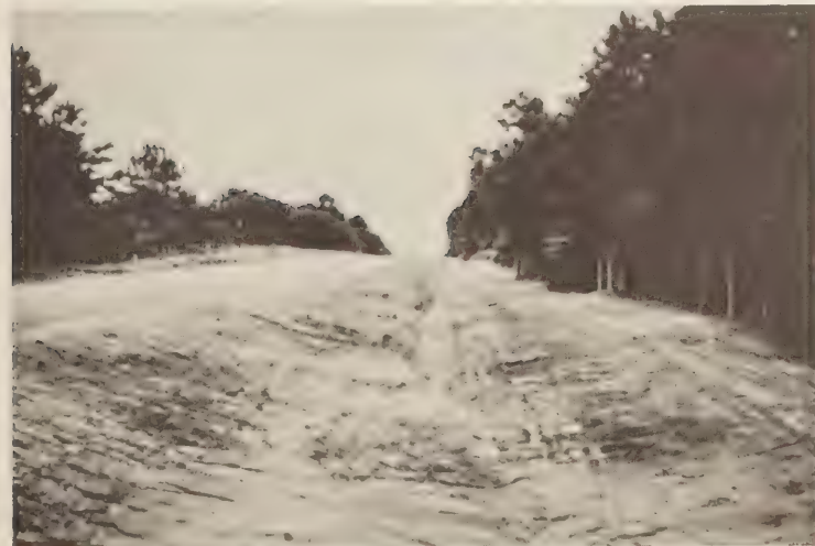
Figure 8.—Ditch graded for placing of roving material.
