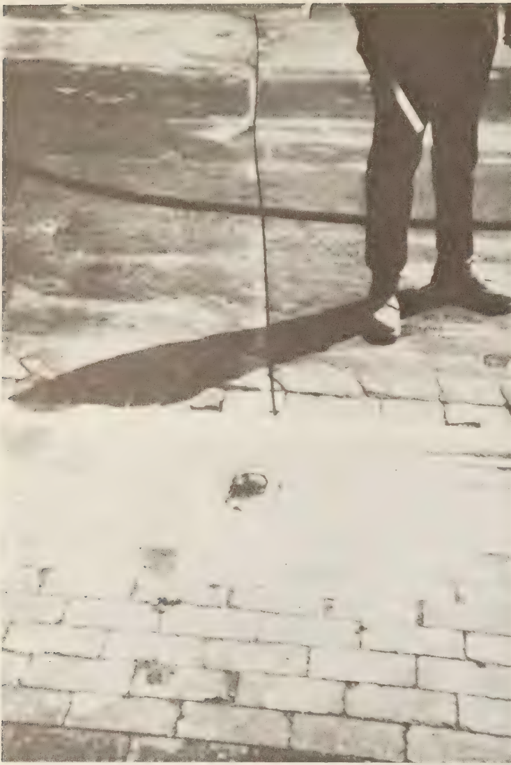
Figure 22.—Finished installation of splice box.
