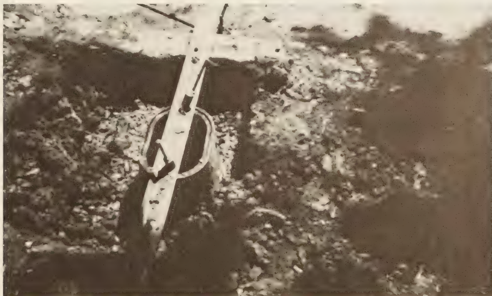
Figure 21.—Concrete around splice box.
