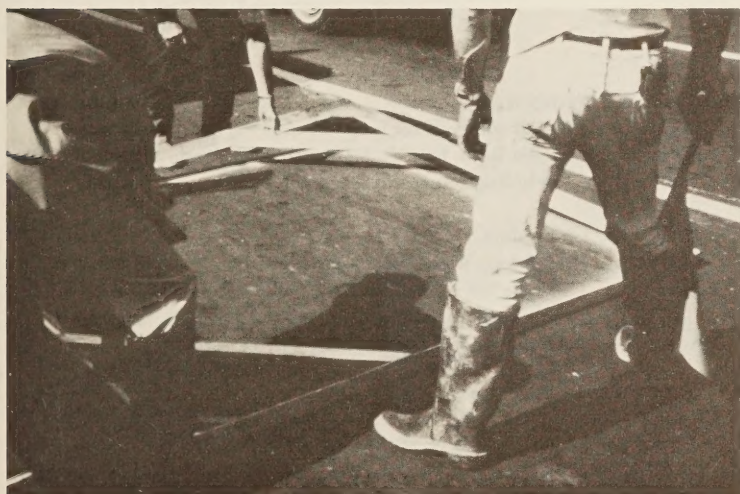
Figure 5.—Template for layout of loop detector.
