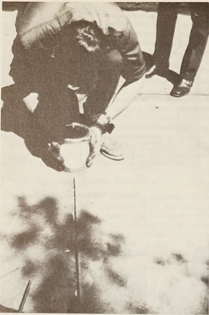
Figure 9.—Placing sealer in slot.
