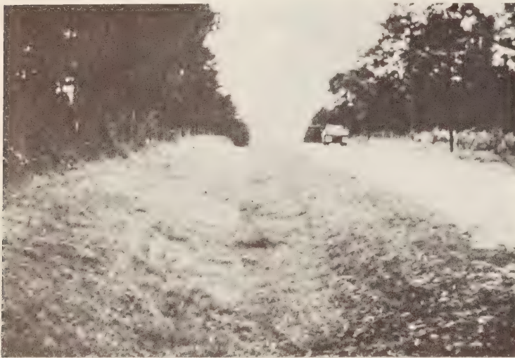
Figure 10.—Restored ditch with grass cover.
