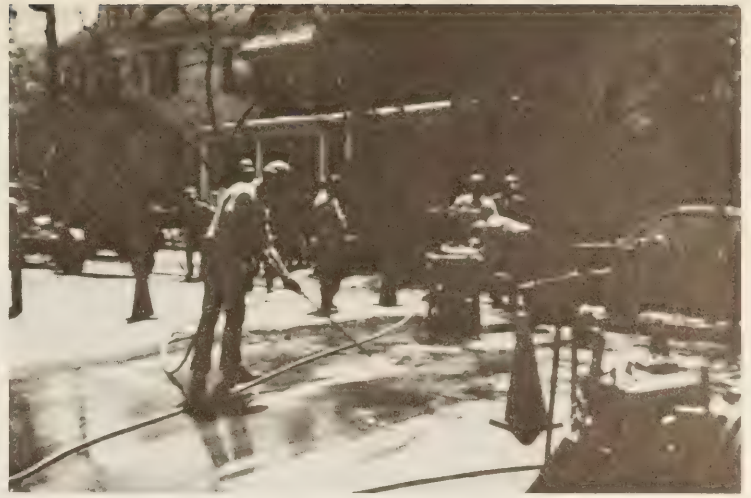
Figure 18.—Cleaning out sawed slots.
