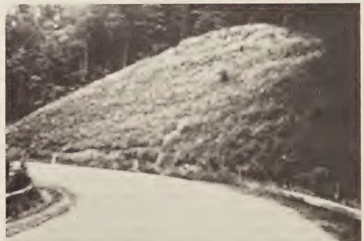
Figure 3.—Stepped slope with gradually disappearing serrations.
