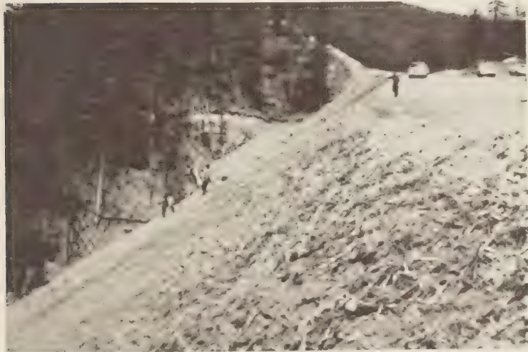
Figure 6.—Wood chips placed on slope in 2-inch layers.
