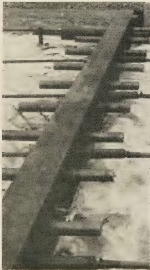
Figure 9.—Closeup of the I-beam which serves as a bearing plate and as support for the dowels. The polypropylene strands pass through metal sleeves.
