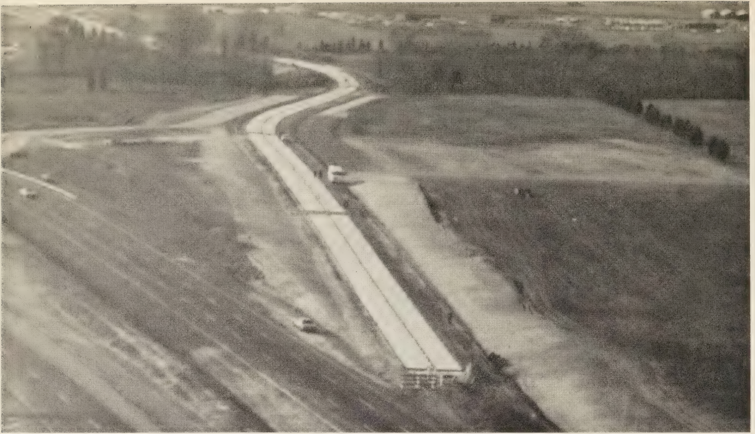
Aerial view, looking east, of the prestressed pavement.
