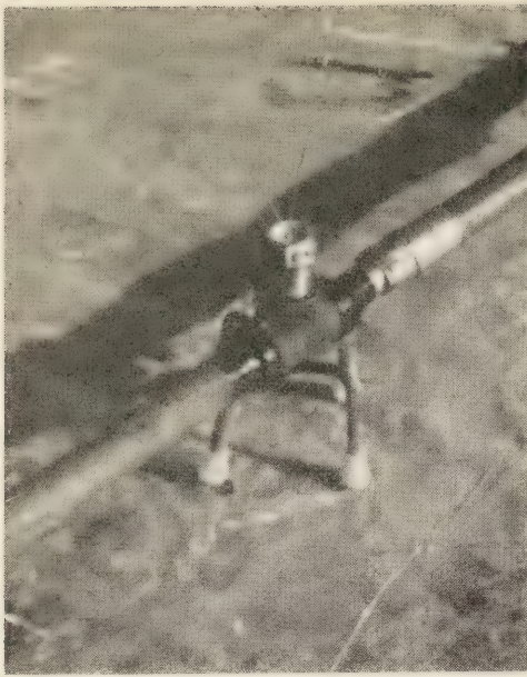
Figure 7.—Closeup of a grout fitting with locating wires projecting from the cap. Grout inlet is \frac{1}{2} inch.
