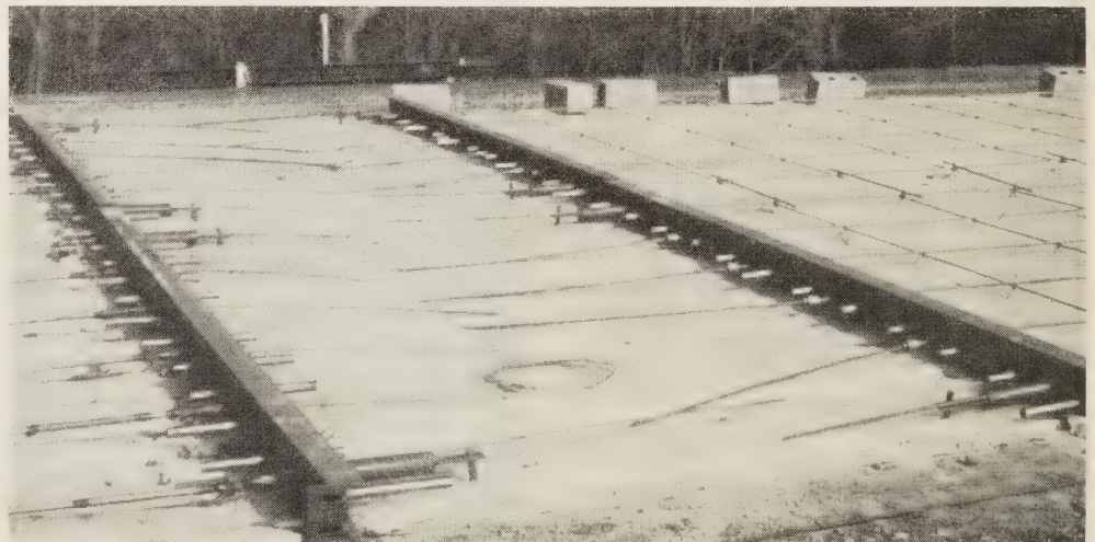
Figure 8.—Joint area between prestressed slabs. An 8-foot-long wire fabric reinforced slab will be placed. I-beams will form the reinforced edges of the 8-foot slab.
