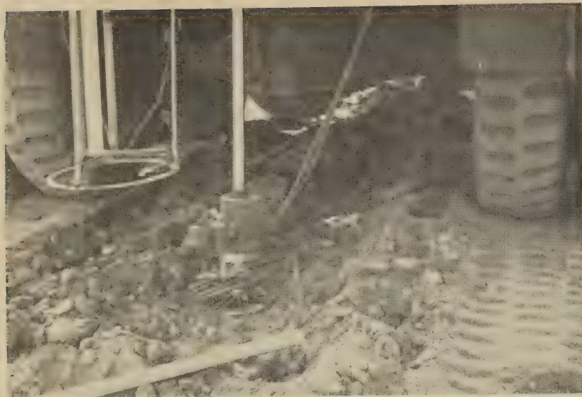
Rapid testing on 6-inch silty-gravel compacted base course. Above left—Plate-bearing test using truck-mounted, hydraulically actuated equipment. Above right—Refraction seismographic test.
