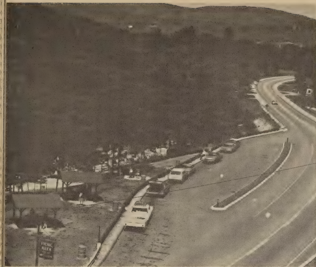
Figure 5.—Snow Falls rest area on Route 26, West Paris, Maine.
