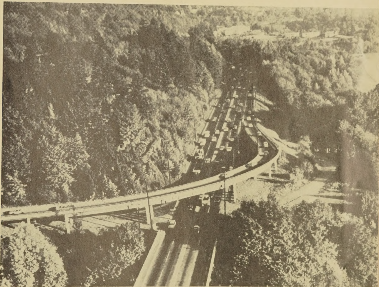
Overhead ramp from Slavin Road to Barbur Boulevard, Portland, Oreg.
