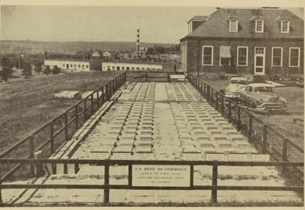
Exposure plot used to test durability of concrete specimens at the Bureau of Public Roads Laboratory
