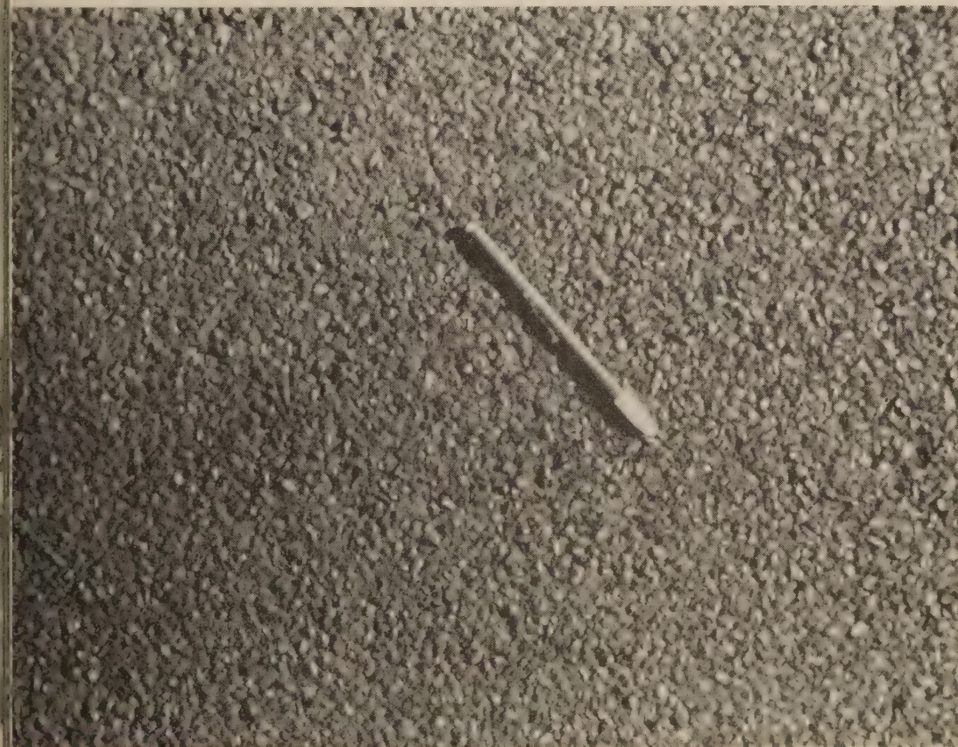
Figure 3.—Close-up of plant-mixed seal coat.
