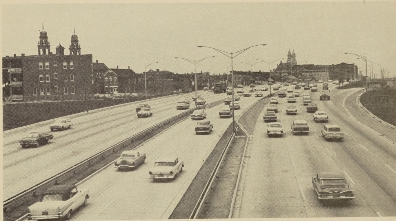
Northwest Expressway, Interstate Route 94. This view, west from Augusta Blvd., Chicago, Ill., shows a section of the reversible roadway for six lanes of traffic and the median shoulders for emergency parking.
