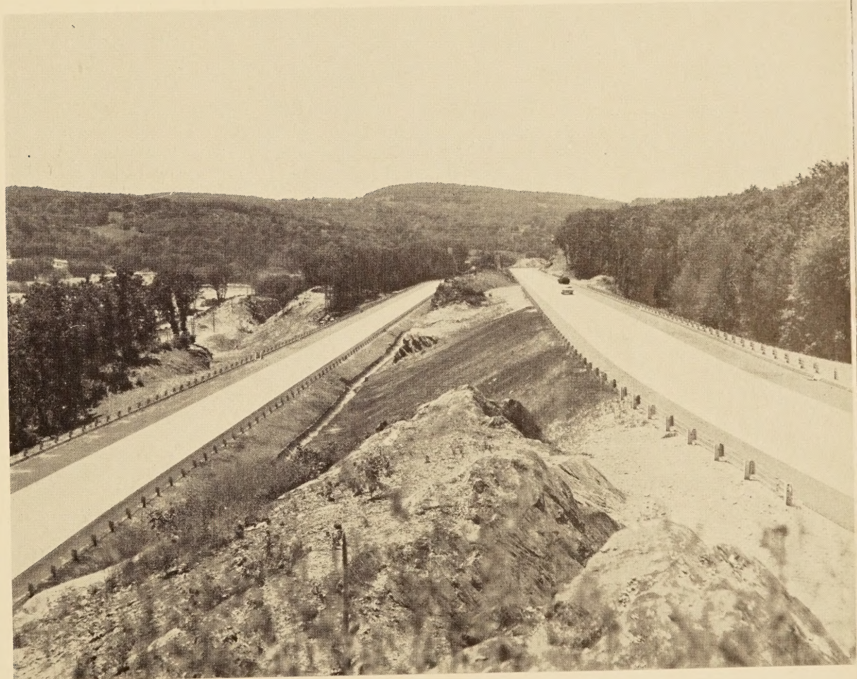
Newly constructed Connecticut Route 8, a Federal-aid primary facility, north of Waterbury.
