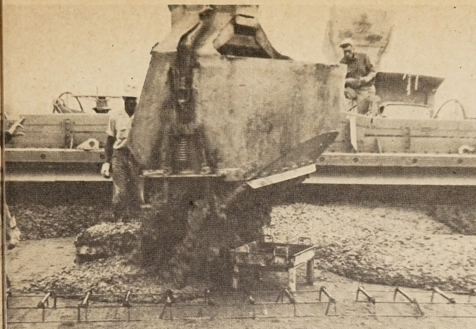
Figure 1.—One of the methods used in obtaining sample concrete.
