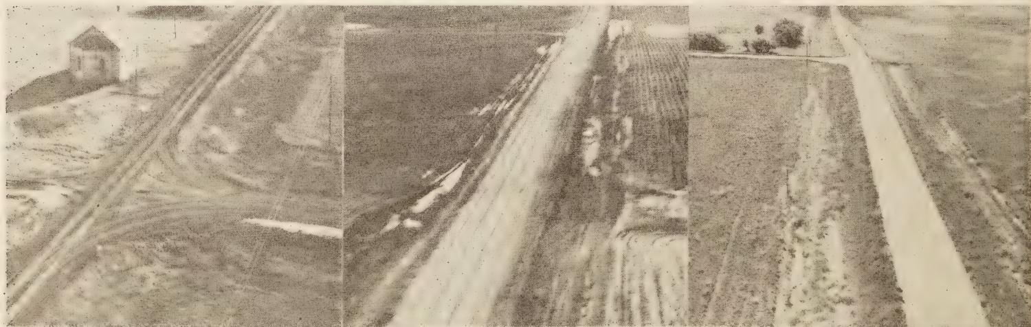
Figure 1.—Aerial classification of low type or unsurfaced road widths: (left) narrow class, single pair of tracks; (center) middle class, three tracks; and (right) wide class, two pairs of tracks.
