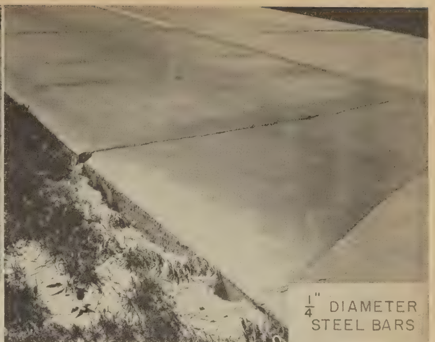
Figure 9.—Cracks at which the reinforcing steel failed. Steel failures in the heavily traveled lane were generally followed by pumping and faulting.
