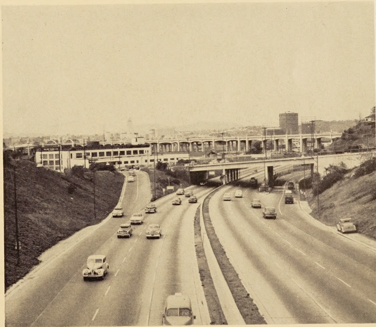
The Santa Ana Freeway in Los Angeles, California
