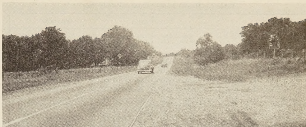
Figure 2.—No passing zone at site N, marked with the national standard, starts near foot of grade in background.
