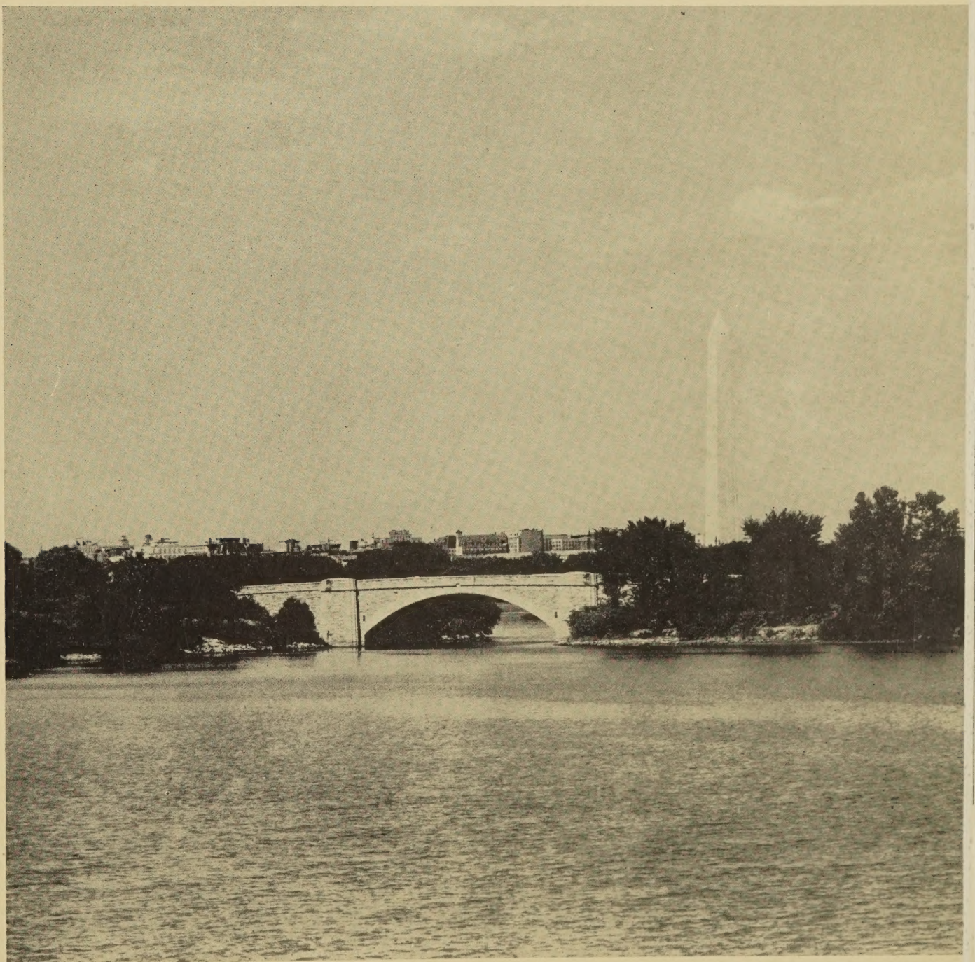
Boundary Channel Bridge, Washington, D. C.
