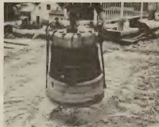
Figure 4.—"Jumping frog" used to compact cohesionless sand.
