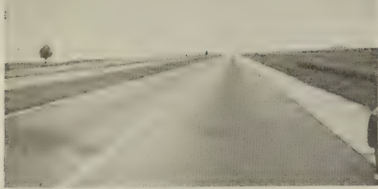
Figure 6.—Where dark-colored pavement was used, the shoulder strips were of plain concrete for contrast.
