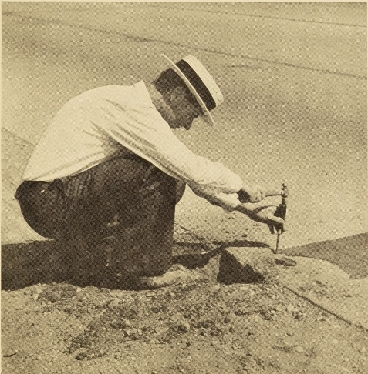
STUDYING JOINTS IN CONCRETE PAVEMENT
