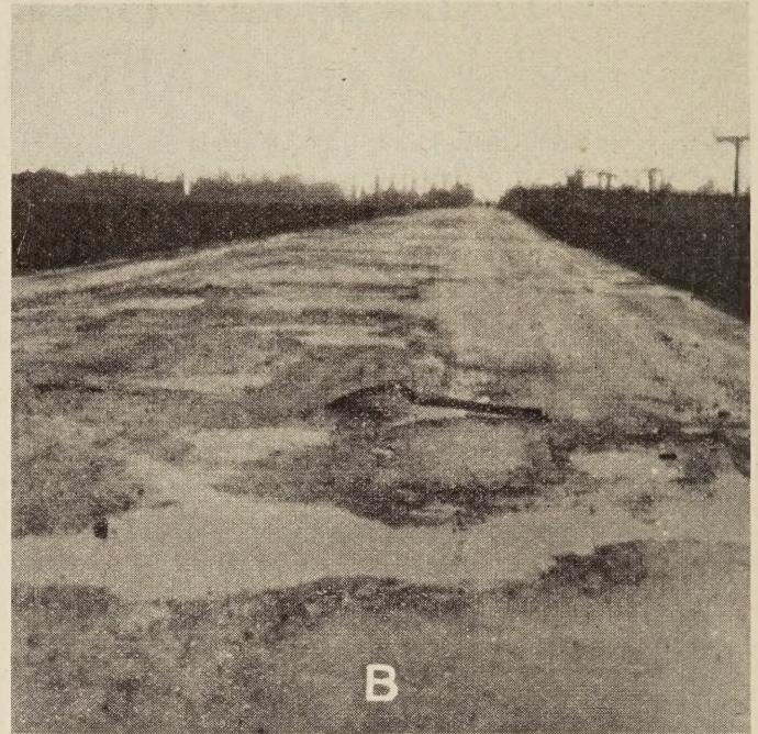
Figure 2.—CONDITION OF OLD BITUMINOUS MAT, A, TYPICAL OF BETTER PORTIONS OF THE PROJECT AND B, TYPICAL OF SECTIONS WHERE SURFACING WAS COMPLETELY DESTROYED.
