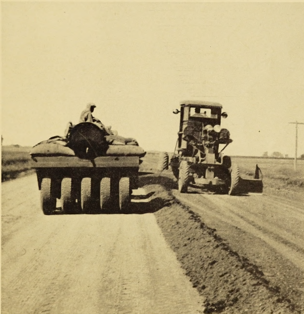
CONSTRUCTING A STABILIZED SOIL BASE
