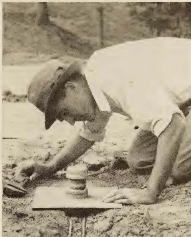
FIGURE 31.—PLACING SETTLEMENT CELL IN OHIO.
